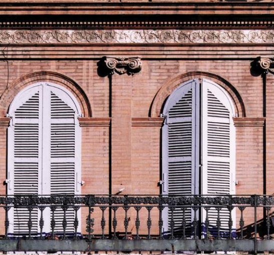
Detail of facade features, Côte des Bonnetiers.
