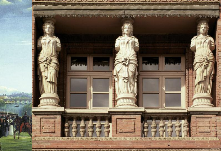
Facade of the former Post Office. A proliferation of moulded brick decorations appeared throughout the 19th century, under the impetus of the Toulouse-based Virebent factory.
