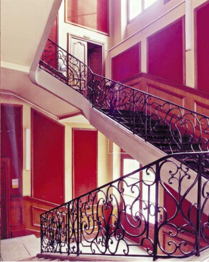
The first steps of the town hall's grand staircase are made of stone, followed by wood for the upper floors in order to lighten the overall structure. A wrought iron banister runs throughout.
